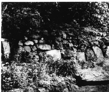
Poolhouse Existing stone wall
